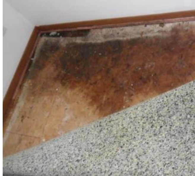
Leak Under The Floor
