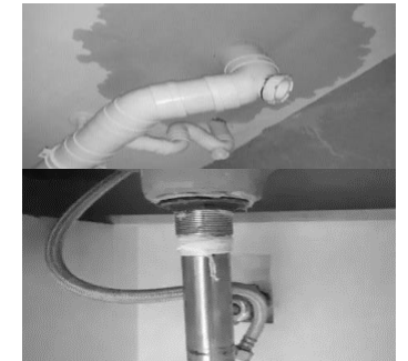
Water Supply Pipe Leakage/ Water Pipe Leakage
