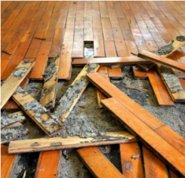
Leak Under The Floor
